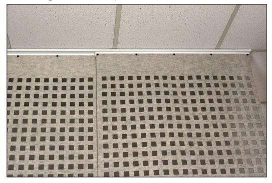
1. Establish the location of the track system. If needed, draw a line to ensure the track will be straight. In our example, we are using the metal railing of the drop ceiling.
