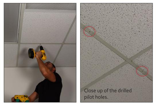
3. **Place the anchors** using an appropriate screw for the surface. After the anchors are in place, pivot them so that the are facing out so the track can fit over the locking mechanism.
