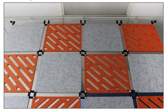
Shown below are the components that will be provided to install the bar for the Modular Panels. Depending on the length of the bar, the number J shaped brackets will vary.
