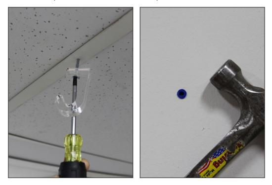
3. After installing all the brackets, insure that they are all facing outward. You can finish by placing the rod and assembled Modular Panels on the brackets.
